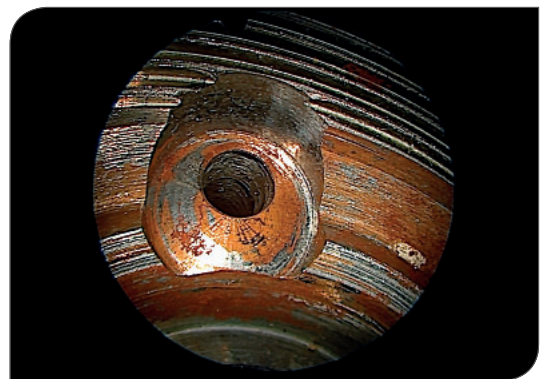
Inspection for wear and corrosion in maintenance
